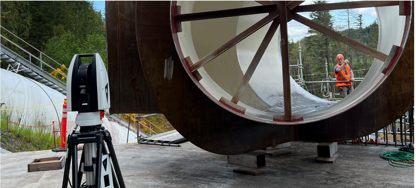
Penstock bifurcation installation
